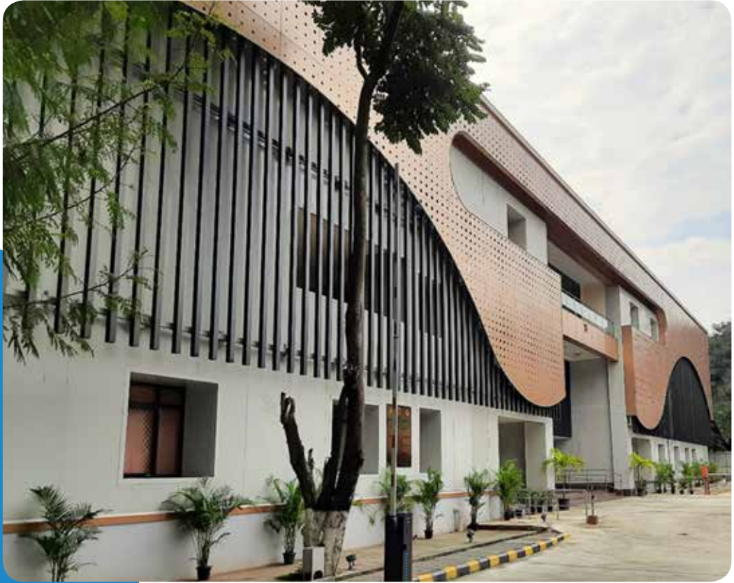
NETRA Building ISTRAC Campus, Bengaluru
