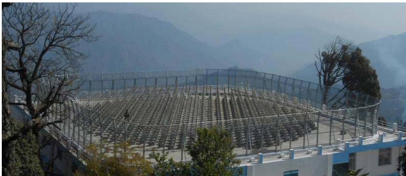
Fig. 2: Recently installed a clutter fence along the periphery of the ST Radar antenna array on the rooftop of the building.
