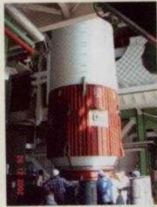
Positioning of NES+CBS module on pedestal
