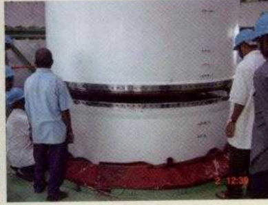
S139 segment joining
