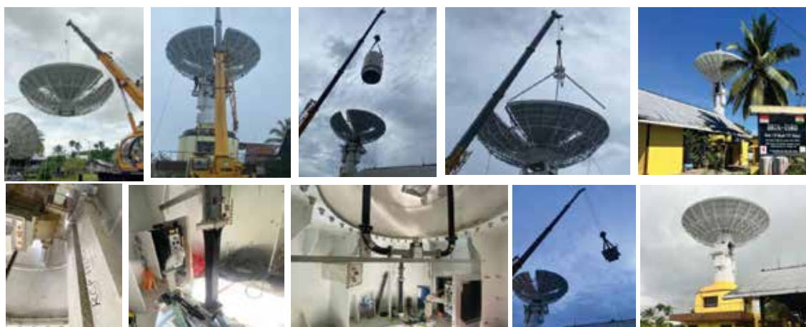
Progress of activities for 11 m Antenna Installation at Biak
