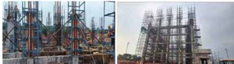
SSLV Launch Pad Construction
