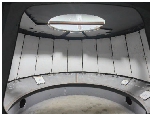
CTS Structure Inner view with Decks assembled
