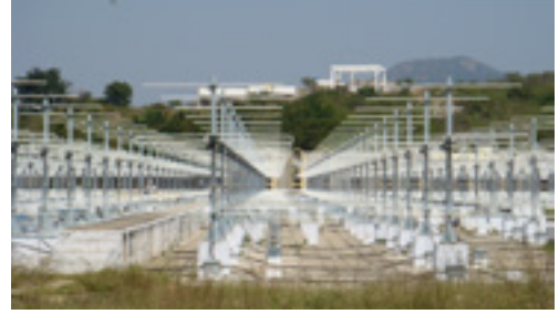
MST Radar Facility at NARL
