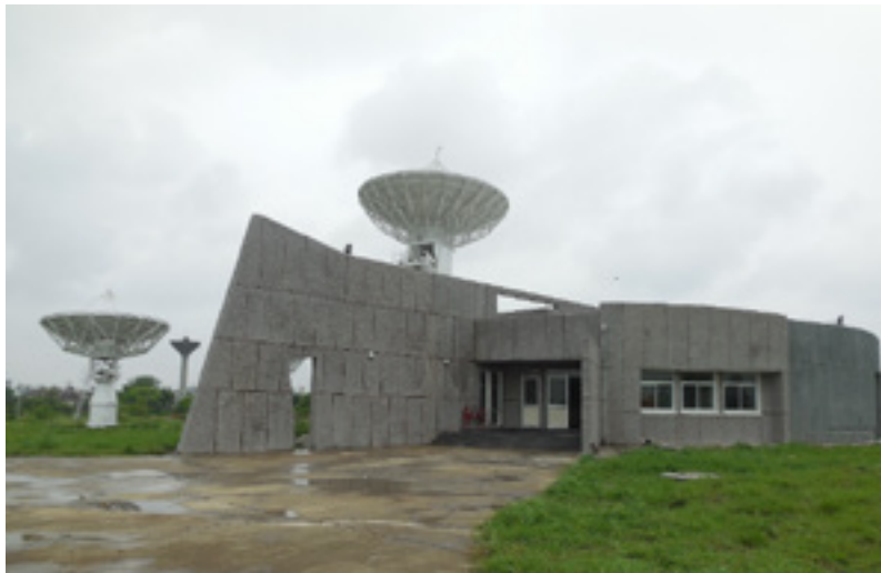
Satellite Control Earth Station with Full Motion Antennae at MCF, Bhopal
